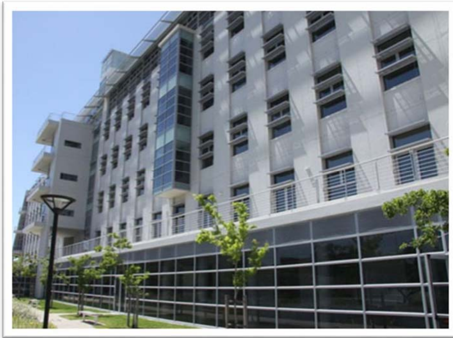
Life Sciences Facility, University of the Western Cape, Cape Town, South Africa
